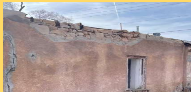
Photos showing flat roof over Back Room (#4) and Bathroom (#5)
