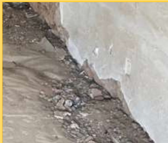
Photos of base of exterior walls, taken from inside of the Stone House. Hand excavation in several locations underneath walls did not discover a foundation
