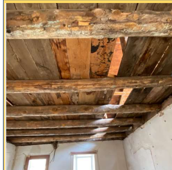
Much of the ceiling has old pine planks above the vigas and timbers.
