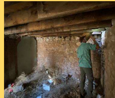
Basement walls are stone and appear to be stable. Some grouting may be required to ensure stability.
