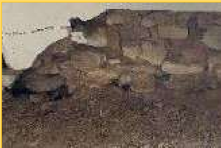
Photos of base of exterior walls, taken from inside of the Stone House. Hand excavation in several locations underneath walls did not discover a foundation
