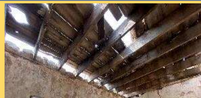
Sawn timbers and 1X comprise the roof structure over these rooms.
