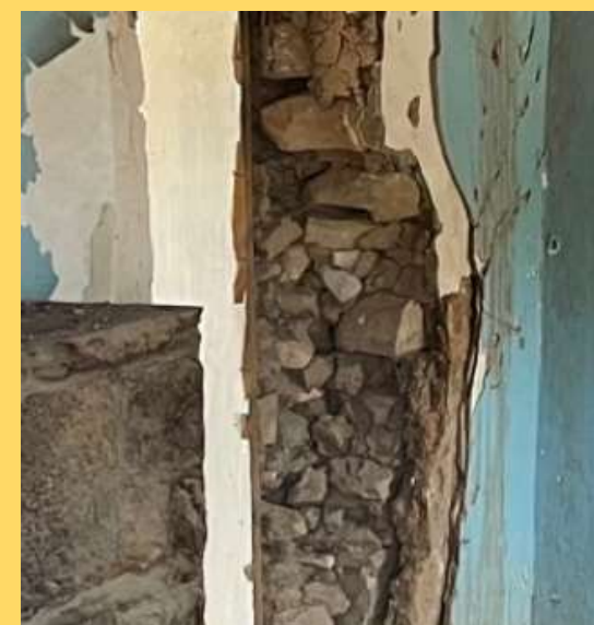
Photos taken inside Back Room (#1). This exposed wall provides a cross sectional view of rock wall construction.
