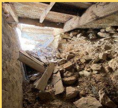
A chute from the room above
