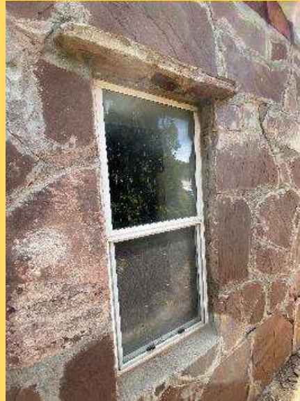
Some windows have been replaced, while some of the old wood frame windows remain.
