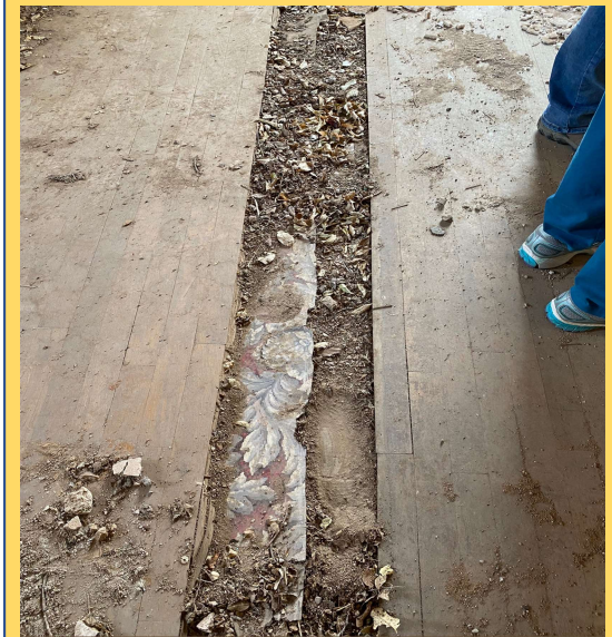
T&G Wood floor in Middle Room (#2)
