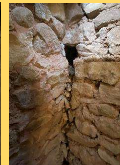
Basement walls are stone and appear to be stable. Some grouting may be required to ensure stability.
