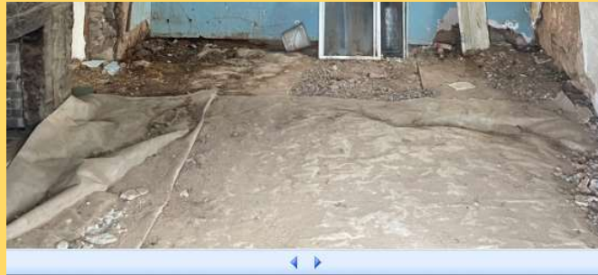
Plastic covers the dirt in Main Room (#1)
