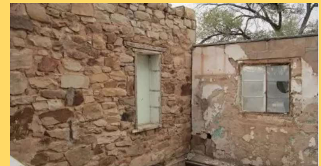
Picture taken from inside Back Room 1 looking North East
