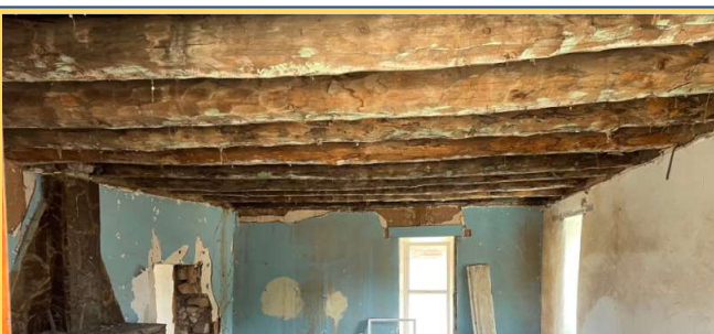
Round vigas of varying sizes are part of the roof structure.
