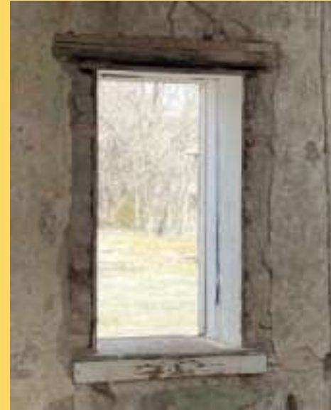
Some windows have been replaced, while some of the old wood frame windows remain.
