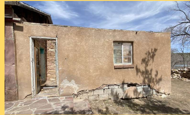
South facing side of Back Room 1 (#3)
