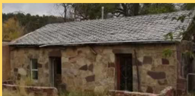
Photos showing pitched roof over Main Room (#1) and Middle Room (#2)
